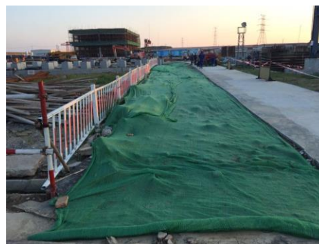
厂区密目网苫盖
