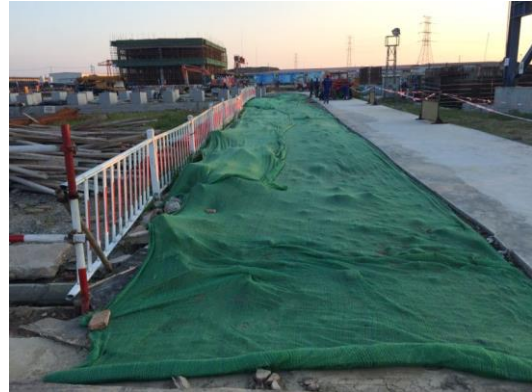
厂区密目网苫盖
